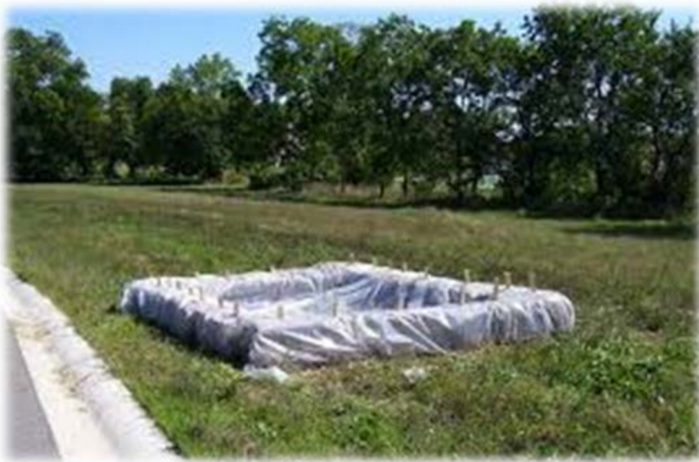
Temporary concrete wash out site preventing contaminants from entering the ground and the storm system.
